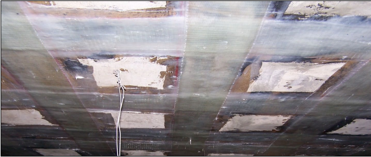
Underside of Slab that is Reinforced with GFRP Strips
