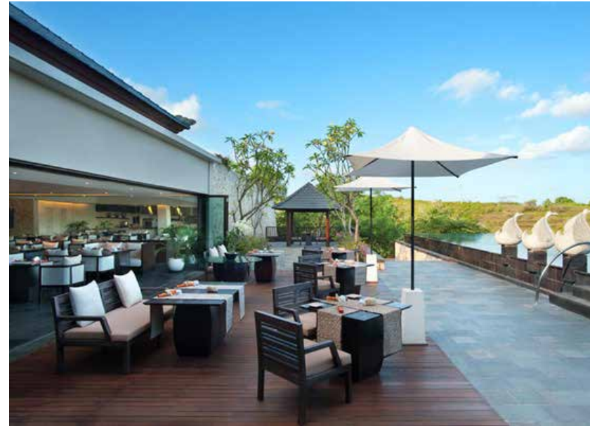
flush set wood decking
