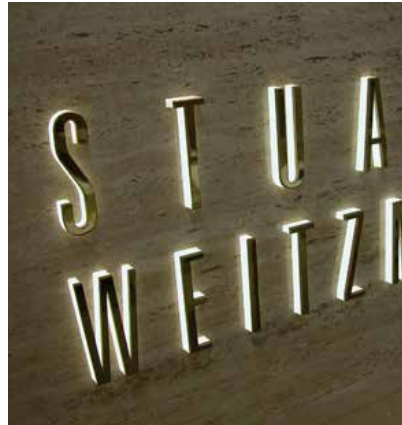
Wall Mounted Sign: Push-through Acrylic letters
