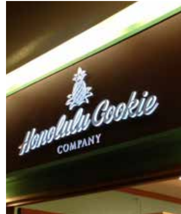
Wall Mounted Sign: Push-through acrylic letters with opaque faces
